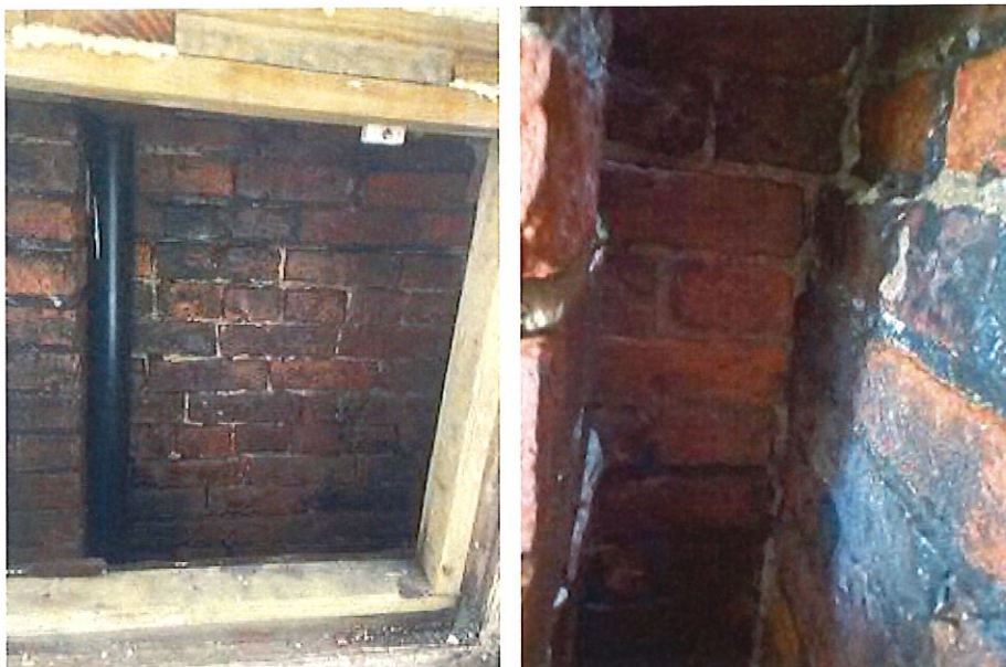
Inspection shaft from Town Hall Yard property
